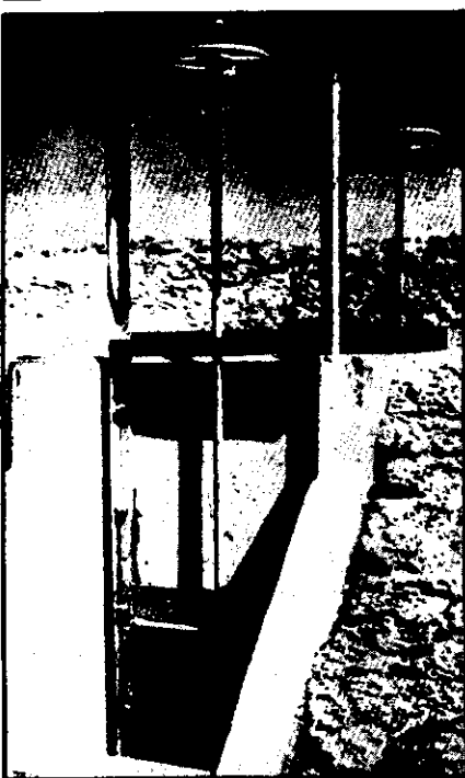
Constant-head orifice turnout inlet.
