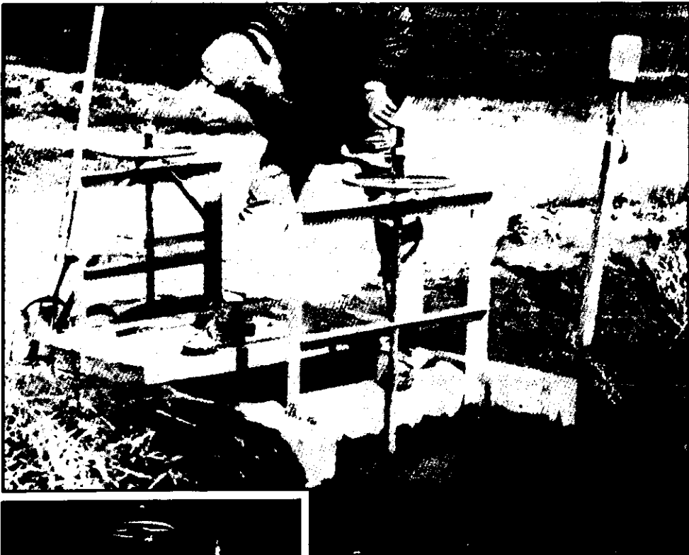
Operator adjusting orifice gate on a constant-head orifice turnout.
