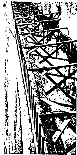
ပုံ 5.4 Elevated flume crossing natural drainage. PX-D-4592
