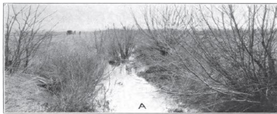
Figure 4 n = 0.080 Dredge channel in black slippery clay and gray silty clay loam, irregular wide slopes and bottom, covered with dense growth of bushy willow, some in bottom; remainder of both slopes covered with weeds
