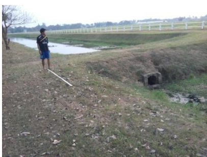
Figure 1 Drainage Ditch D3-SD
