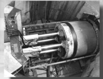
A construction of ID 3-m Main Trunk by pipe-jacking Method ▼
