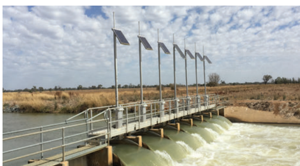
c. Multibay flumegate regulator, Macalister Irrigation District (Source: Southern Rural Water)
