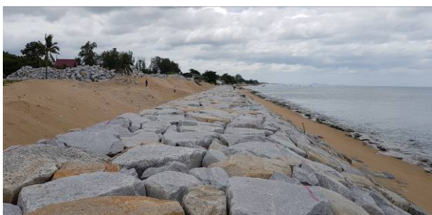
Fig. 8. The seawall was under construction along Ban Thung Pradu.
