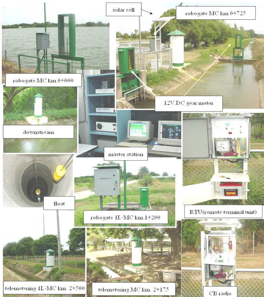
Figure 2: Photo of Kamphaengsaen canal automation system
