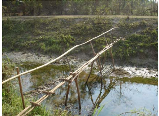
Bridge for flow measurement at main canal
