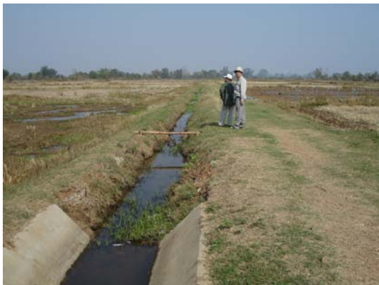
Bridge for flow measurement at tertiary canal
