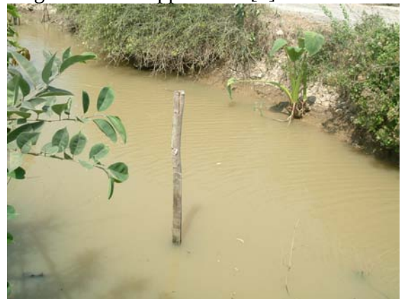
Staff gauge installation for monitoring water level changes in canal or changing of dept lifted by pump
