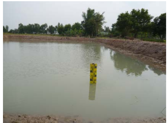
Percolation in fishpond
