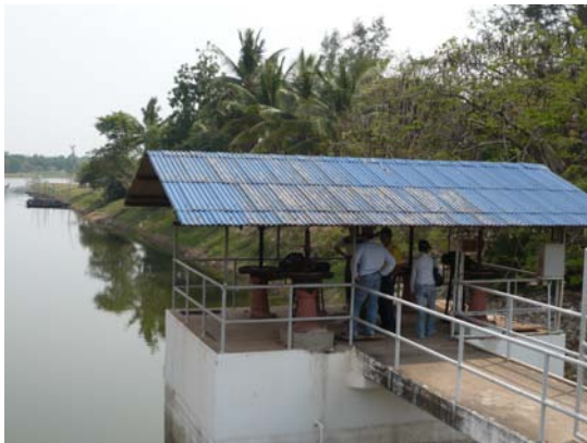
Checking gate operation at inlet of main canal
