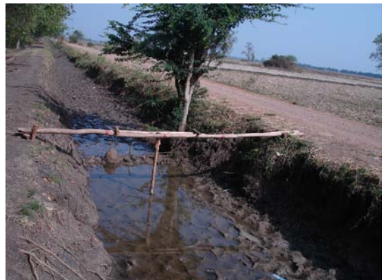
Bridge for flow measurement at secondary canal
