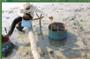
Installation of evaporation tank
