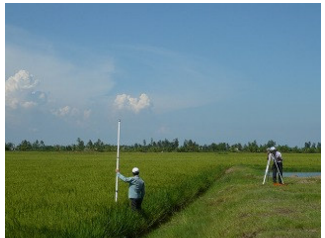
Ckecking level of satffguage installation
