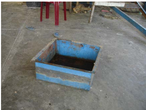
Small evaporation tank
