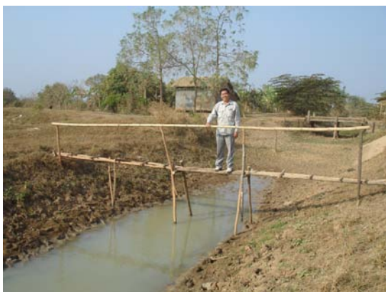
Bridge for flow measurement at drainage canal
