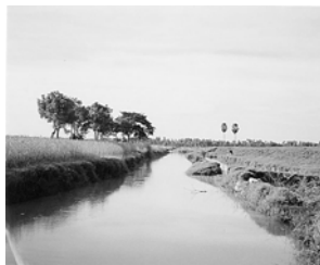
Existing Main Canal
