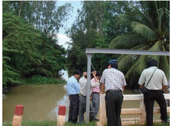
Observing HL 6 sluice
