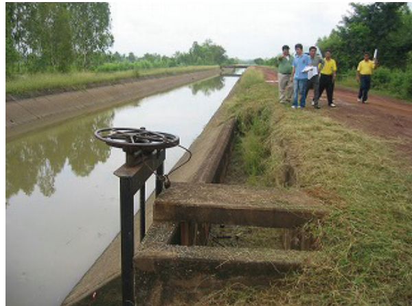
Observing irrigation structure
