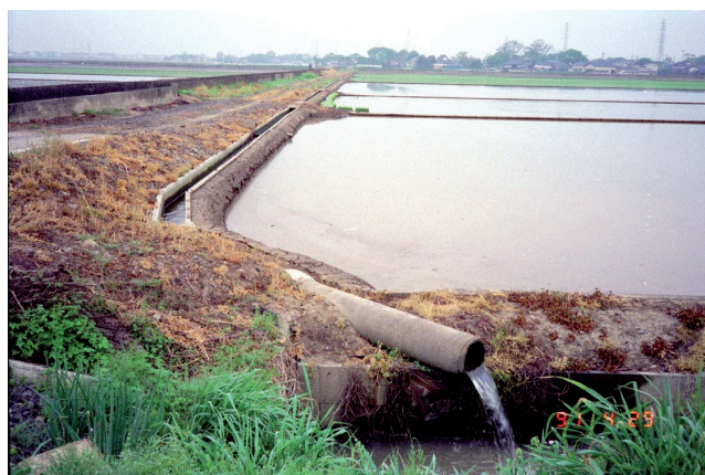
Figure 3.8 Overflow from a tertiary canal
