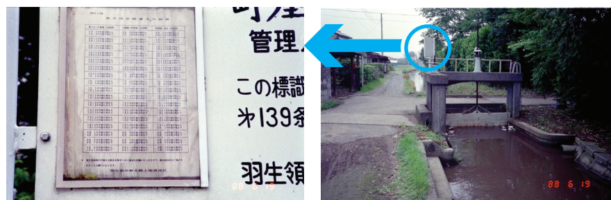
Figure 3.3 Bulletin board informing water users in each sub-irrigation system of the water delivery rotation at irrigation turnouts
