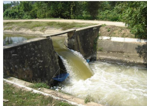
Check Drop with Rectangular Opening (Phetchaburi O&M Project)
