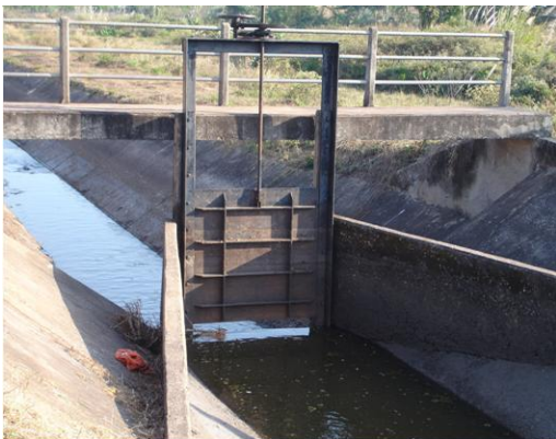
Mixed Regulator for Limited Canal Width Operating in Undershot Mode (Phetchaburi O&M Project)
