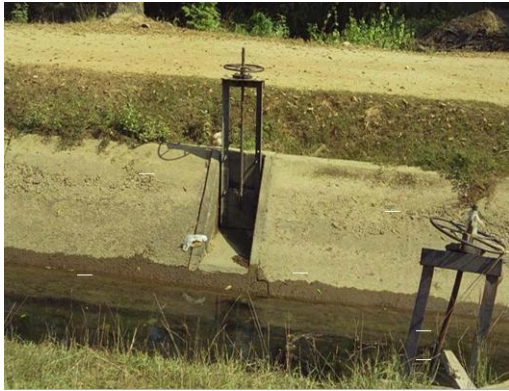
FTO with single gate control (Phetchaburi O&M Project)
