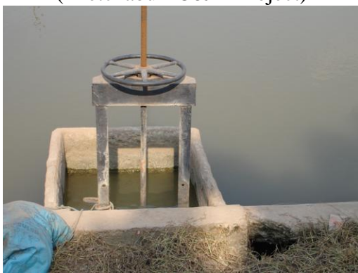
FTO with single gate control (Phetchaburi O&M Project)
