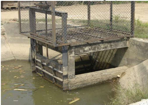
Mixed Regulator for Limited Canal Width Operating in Undershot Mode (Phetchaburi O&M Project)
