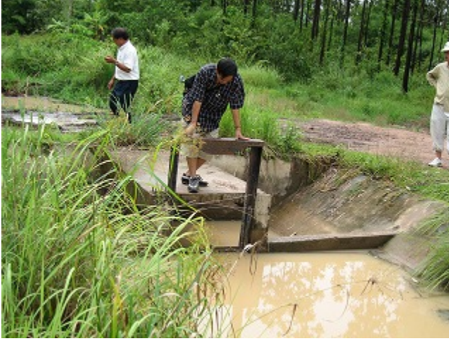
Observation at End-Canal Spill point
