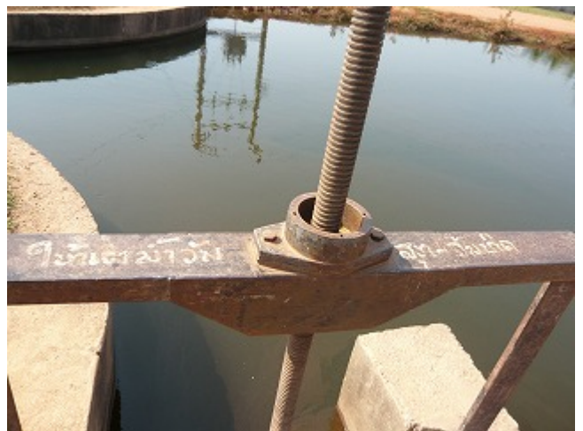
Gate at Canal N4
