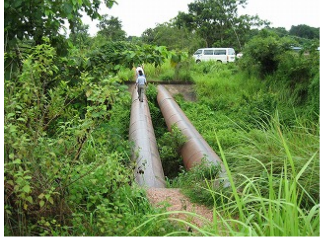
Siphon at Main Canal
