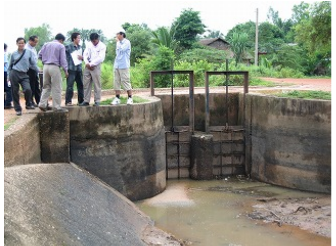
RAP Conducting- Observation of Structures along Main Canal
