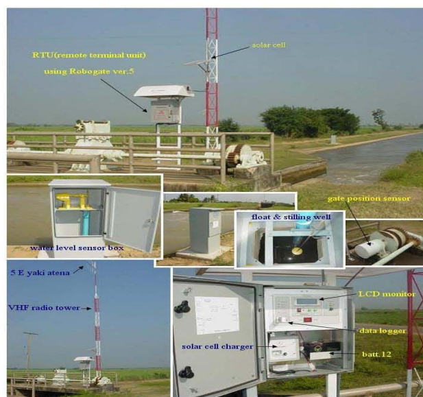
Figure 2 Robogate at Cross- regulator
