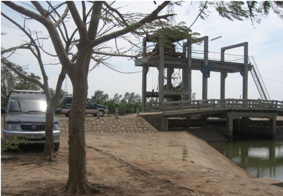
Photo 2: A photo of Longhai sluice
