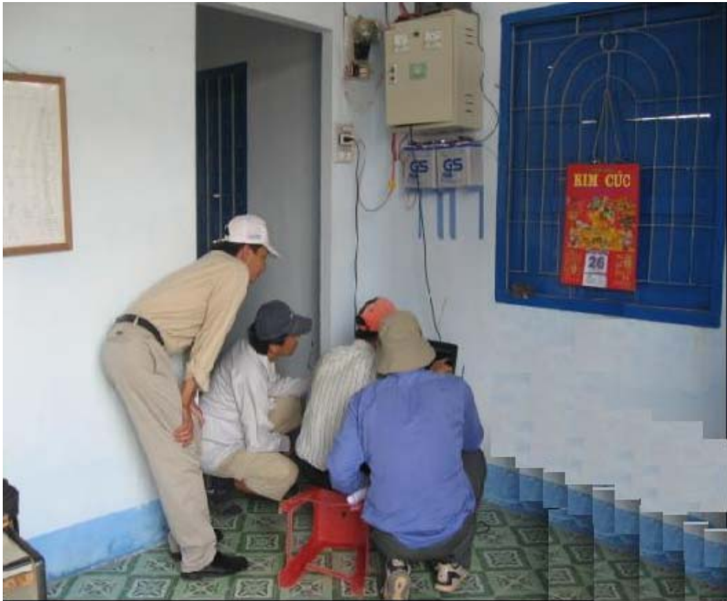
Photo 3: Data downloading from Longhai station
