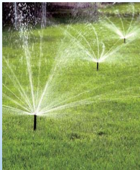
Sprinkler Irrigation ( E_a = 70-80\% )
