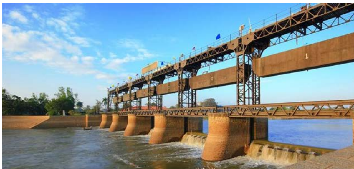
Fig. 9 Rama 6 Barrage in Pasak river, the first river barrage of Thailand
