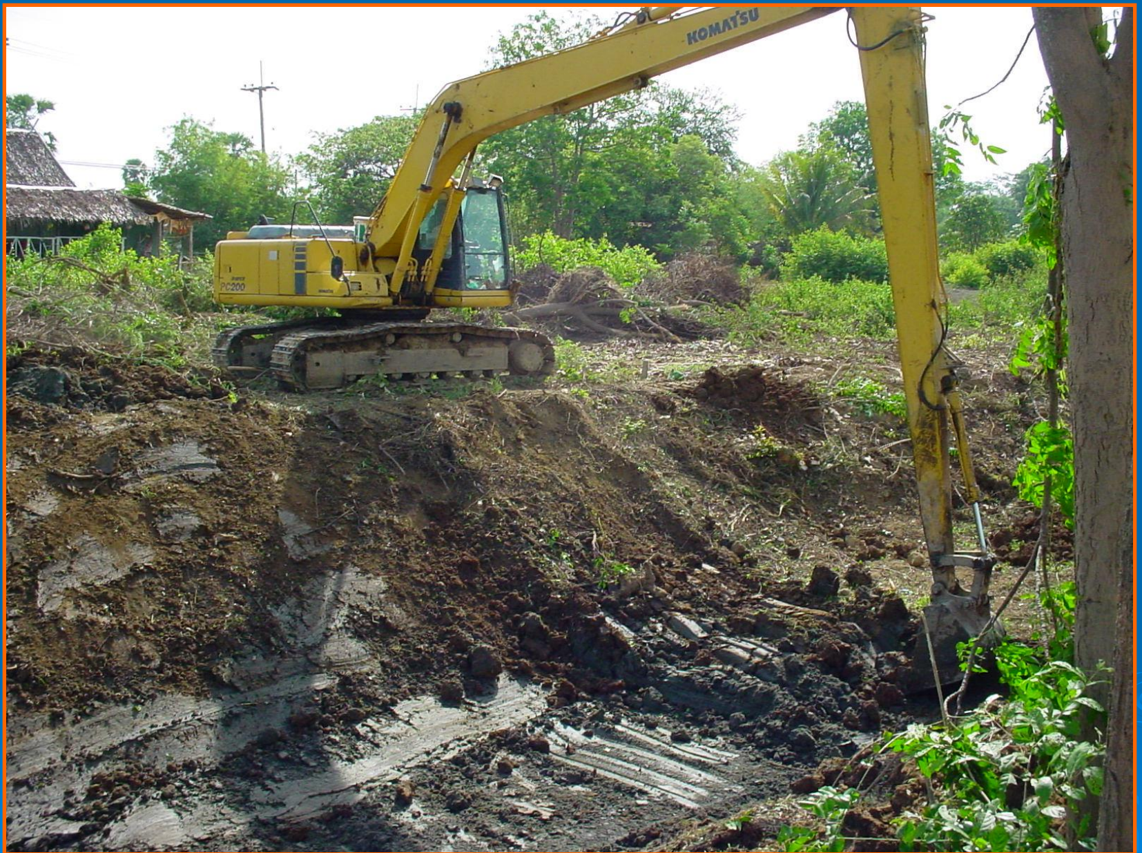
Removal of sediment from stream
