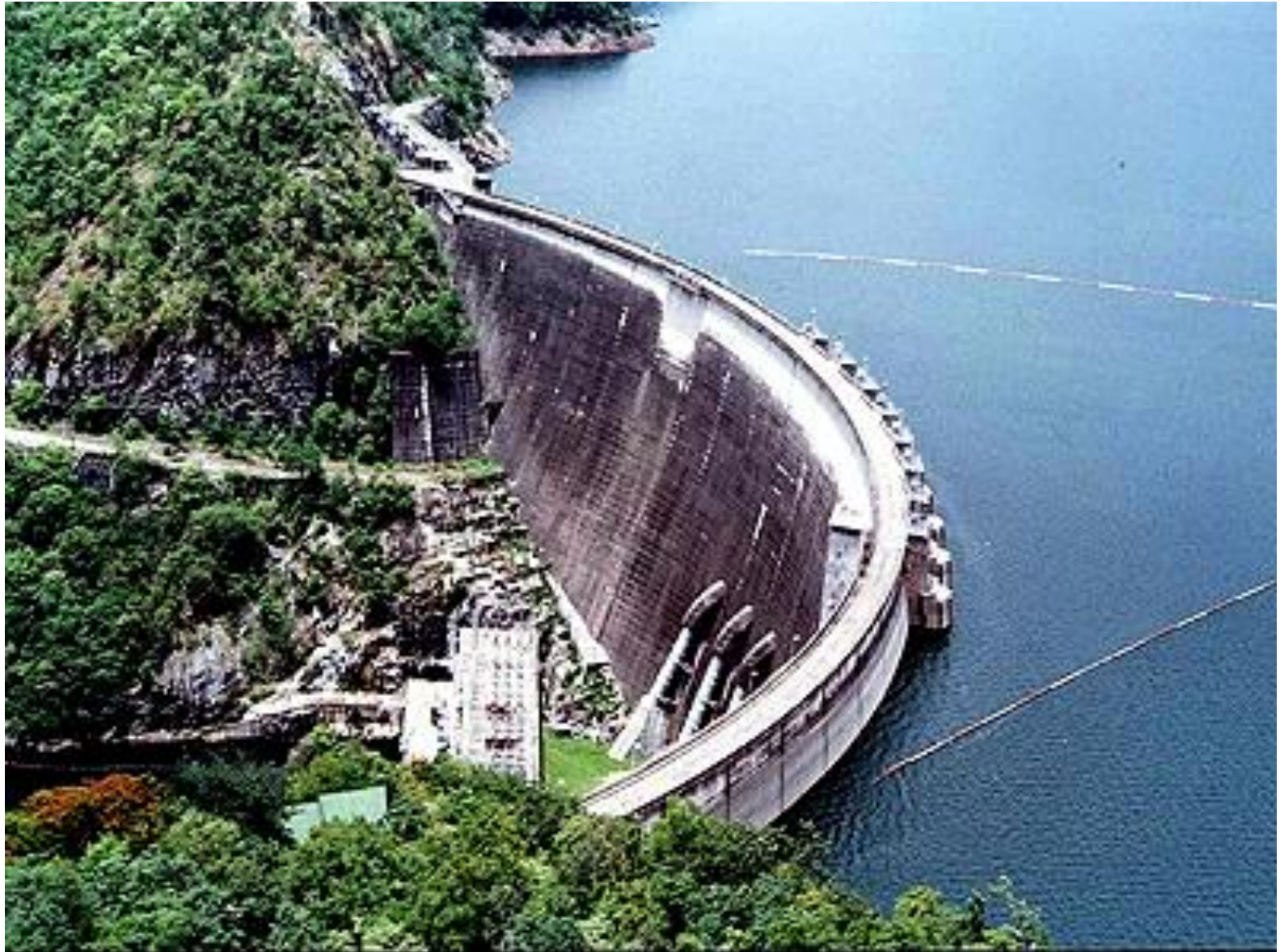
Bhumibol Dam The largest concrete arch dam in Thailand
